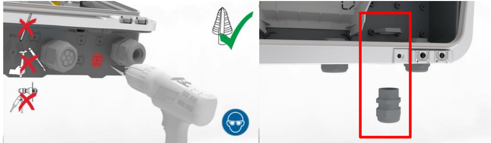
Picture 3: Drilling the base unit and inserting PG-screw connection at the modified area.
